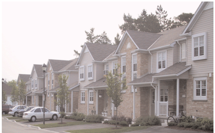
Figure 1: Typical Townhouses at London Lane
