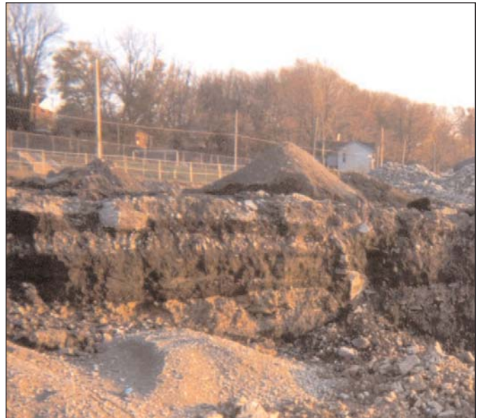
Figure 3: "Black Fill Layer" found during the remediation of the Wellington Square site.
