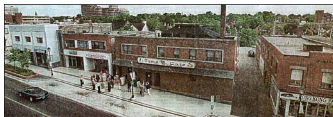
Figure 2: Before photograph showing small businesses on King Street
