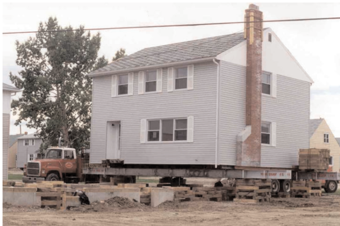
Figure 4: Hundreds of the old houses on the military base were refurbished and relocated at increased densities.
