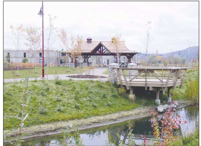
Figure 3: The commemorative structure showing the rejuvenated Brandt’s Creek and a look out.
